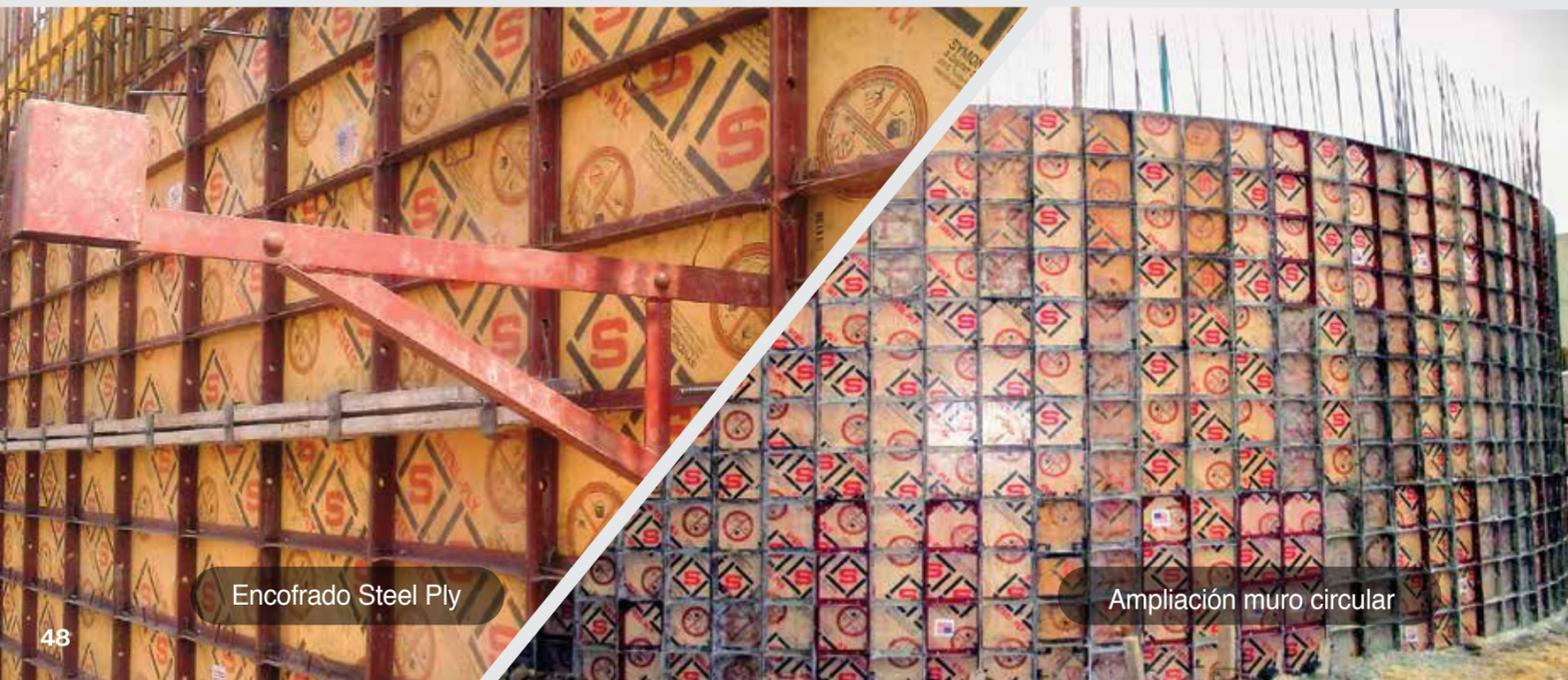
Encofrado Steel Ply
